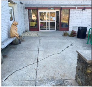
cracked sidewalk
